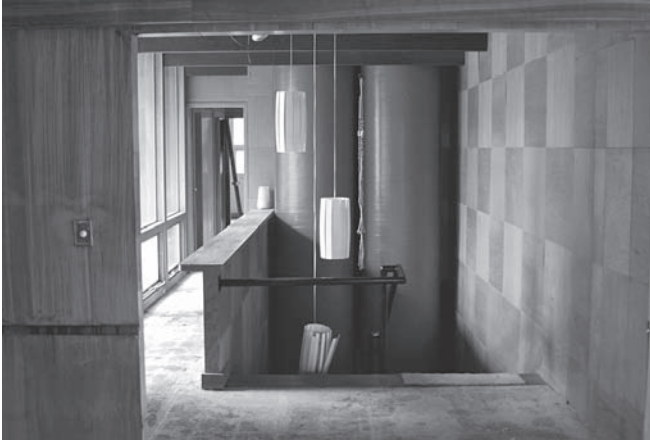
Figure 3. Columns filled with heat-storing river pebbles, in the Löf House. Photograph courtesy Anthony Denzer.
