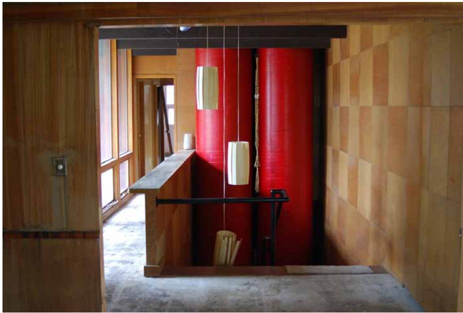
Figure 1 George O. Löf and James Hunter, Löf House, Denver, Colorado, 1957, columns filled with heat-storing river pebbles (photo by Anthony Denzer; used with permission).
